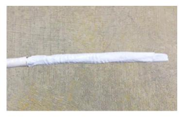
\* Cut binder tape lengthwise with a small scissors
